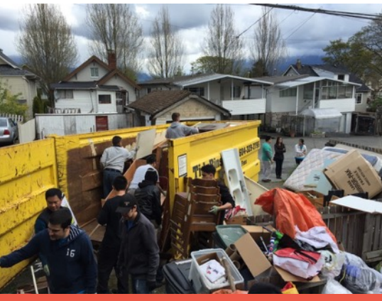
Volunteers helping remove trash from the basement in preparation for renovation.
